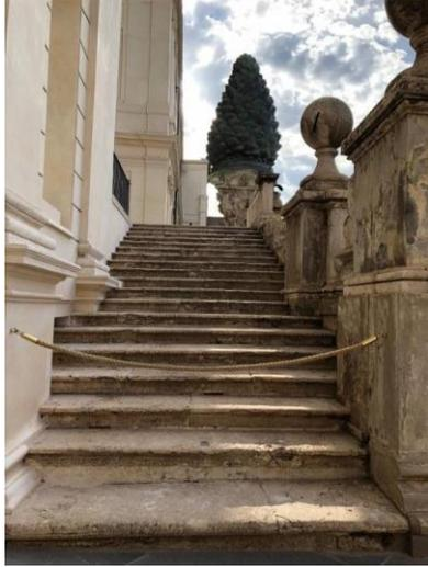
A biocide treatment is being applied on the marble to prevent plants and lichens to grow on the pavement of the terrace and walls. The whole floor will be treated with a special process named “*bocciardatura*” which will allow the marble to retrieve its ancient and beautiful look.
